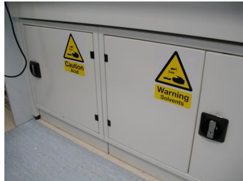
Ventilated Acid and Solvents Store
