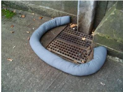
3. Control the spread of the spill by using spillage absorbent granules or other absorbent materials or booms.
