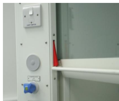
Red tab indicates the Safe Working Limit. But try and work with the sash lower if possible
